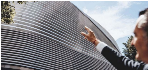
A gleaming stadium: Lasercor cut around half of the almost 9,000 lamellae for the spectacular outer shell of the Bernabéu Stadium in Madrid with millimeter precision.
