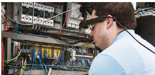
TRUMPF customers in the United States have the option of using smart glasses to speed up repairs when they have a technical problem. Once activated, the glasses automatically film exactly what the customer is looking at and stream the video feed in real time to an experienced service engineer. Like this they can solve the problem together.
