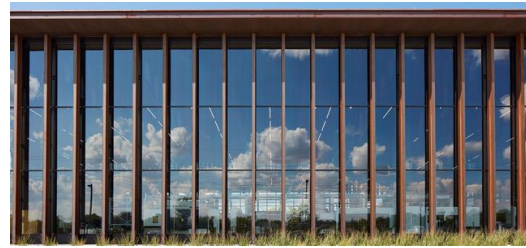
The focus of the Smart Factory is to advise and train customers on the introduction of digitally connected production solutions. Picture: Steve Hall © Hall+Merrick
