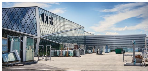
The KFK building in Croatia.
