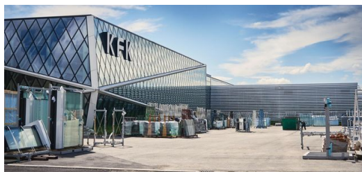
The KFK building in Croatia.
