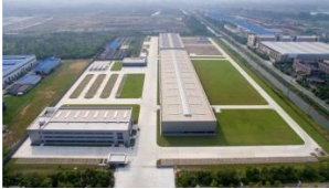
JFY New production facility
