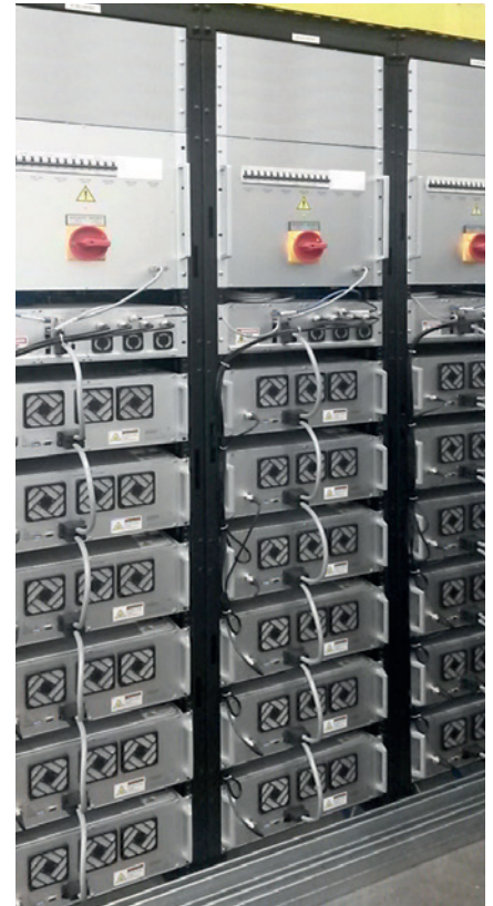
Amplifier 20 kW, 322 MHz
