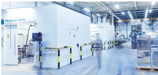
Two laser welding cells connect components to each other. (© Tim van der Most)
