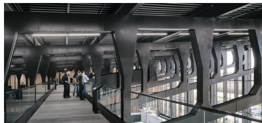
The roof of the production facility at the TRUMPF Smart Factory in Chicago is supported by eleven steel trusses, each made up of many individual
