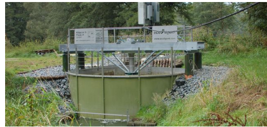
The load-bearing elements of the fish-friendly weir are manufactured entirely on the TruLaser Tube 7000. Picture: Jan Gutzeit
