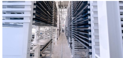
The fully automated Stopa storage system at KNOLL is 70 meters long. It also boasts more than 1,200 storage spaces and 13 loading/unloading stations. Picture: Stephen Duscher
